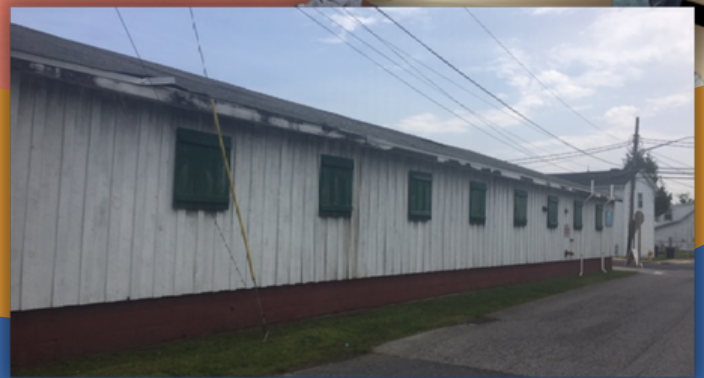
The St. Michaels Community Center prior to renovations.
