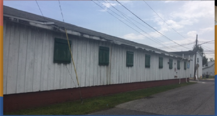
The St. Michaels Community Center prior to renovations.
